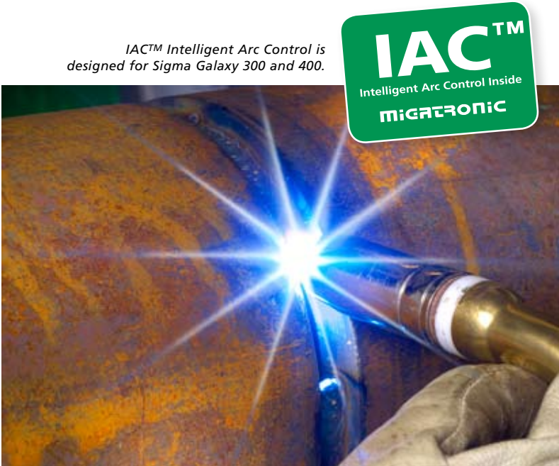
IAC™ - Vertical downwards welding of a root pass in a district heating pipe. Welding speed is significantly increased compared to traditional upwards welding.
